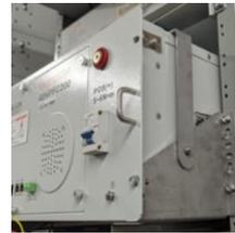
19" Mid-Mount Bracket with support for NPFC200. Shown above is also a 23" extender.
